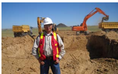
Mining of overburden underway
